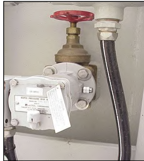
Figure 32 – Photograph of a Sudden Pressure Relay.
