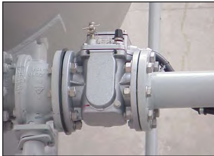
Figure 34 – Photograph of a Buchholz Relay.
