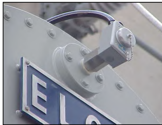
Figure 41 – Photograph of a Bladder Failure Relay.
