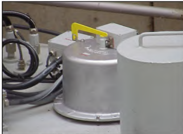
Figure 30 – Photograph of a Pressure Relief Device.
