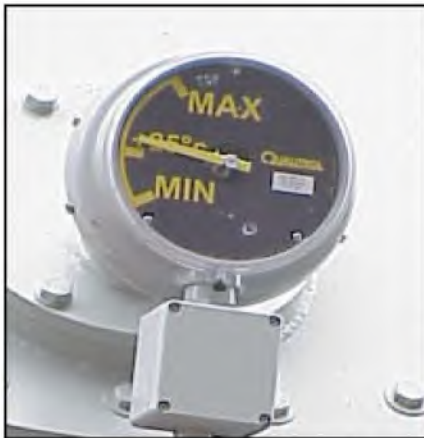
Figure 28 – Conservator Oil Level.
